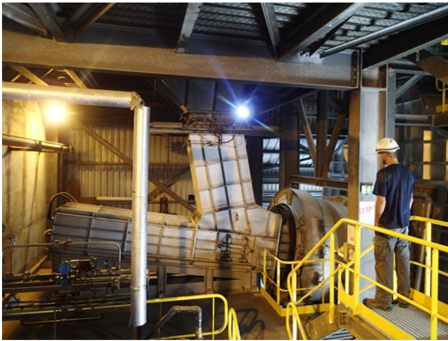
Figure 12. A worker observes operations inside the incinerator facility.
